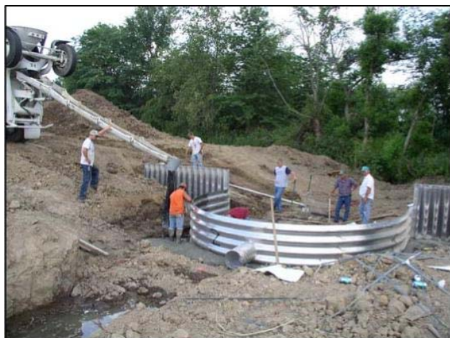
Contractor installing large grade stabilization structure
