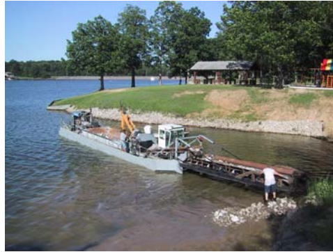
Lake Sara Pilot Site – Barge Laying 1 st Stones
