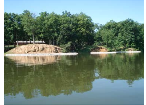
Lake Sara Pilot Site – Finished Transitional Wetland Riprap Breakwaters
