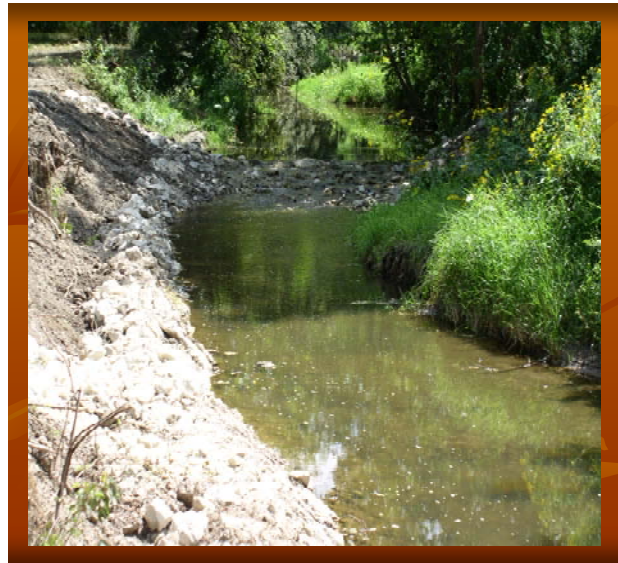
PICTURED ABOVE: Photos of the SSRP site before and after construction. Banks had excessive erosion and we fixed the site with a Rock Riffle and Stone Toe Protection.
