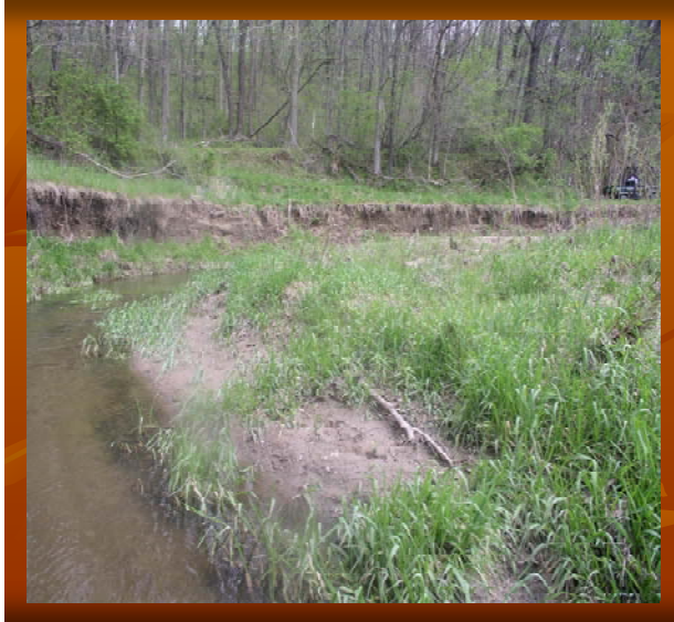
PICTURED ABOVE: Photos of the SSRP site before and after construction. Banks had excessive erosion and we fixed the site with a Rock Riffle and Stone Toe Protection.
