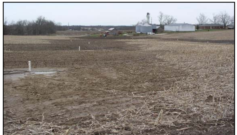
A recently constructed water and sediment control basin system. Cost-share assistance was provided by the district.
