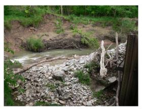
Pictured here is at a concrete structure on Big Creek in Union County. The 13 inch rain created a new channel completely around the structure. Estimated soil loss at this site was more than 3000 tons of soil loss at one time. Estimates to replace the structure was around \$250,000.
