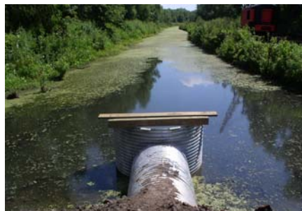
This structure is used to control water levels in a wetland that was added for enhance wildlife benefits for this landowner's CREP enrollment.
