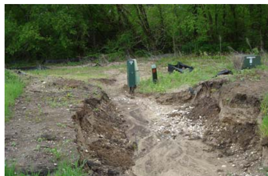
Gully caused by excessive runoff. Notice the high voltage utility box on right side.
