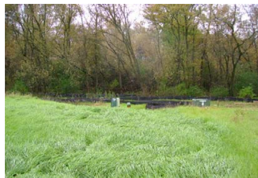
Later in the fall, the same gully has been filled and stabilized with ryegrass.
