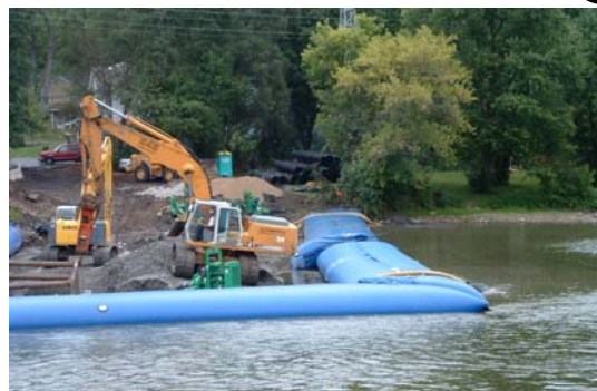
Aqua-Barriers in the Fox River at Batavia help assure an accessible construction site while protecting the river from construction site erosion.
