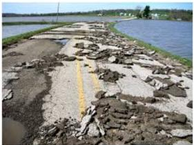
Left: The road has been destroyed by overland flooding resulting from stormwater runoff from impervious and unprotected surfaces. Conservation practices applied to agricultural lands and in urban areas could perhaps have reduced the amount of runoff sufficiently that existing ditches and stormwater conveyances could have saved the road.
