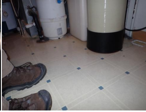
All lines wet from water backup. Leaked on floor by furnace.
