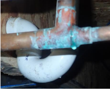
All lines wet from water backup. Leaked on floor by furnace.
