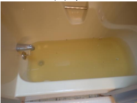
Water had a bad smell and color as it flowed out of the faucets - needs the water purification system updated on maintenance and repaired - change filters and make sure it is working properly.
