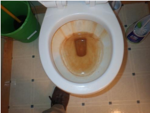
Water had a bad smell and color as it flowed out of the faucets - needs the water purification system updated on maintenance and repaired - change filters and make sure it is working properly.
